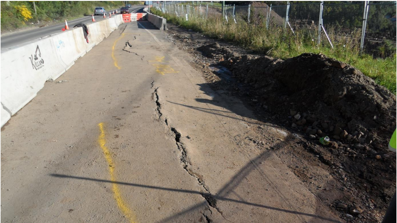
Figure 1: Excessive movement of retaining wall causing road damage and onward failure of water main
